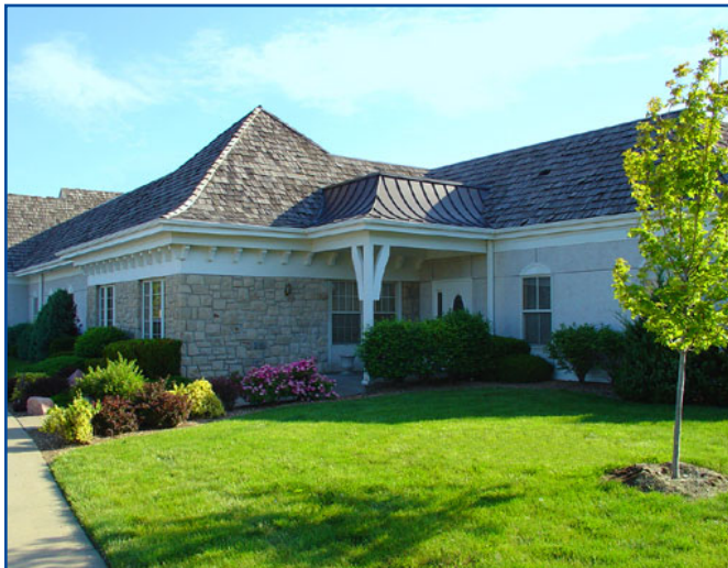
Pictured above is the new ACCP headquarters location in Lenexa, Kansas.
