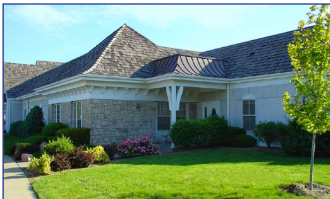
Pictured above is the ACCP headquarters location in suburban Kansas City.
